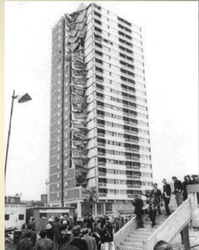
Ronan Point Apartment Tower Collapse London, 1968 wikipedia.org
